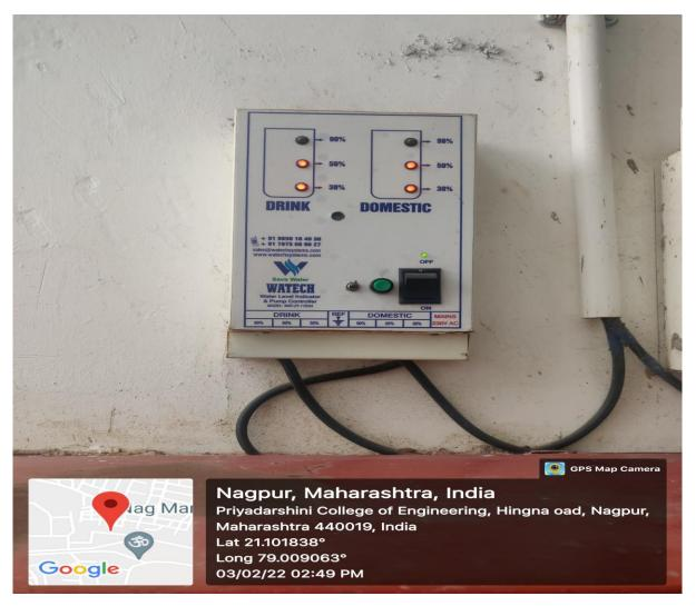
Sensor Based water level controller is installed at ground floor in admin building of PCE which senses the water level in overhead water tank situated at top floor of the building and raises the alarm, accordingly.
